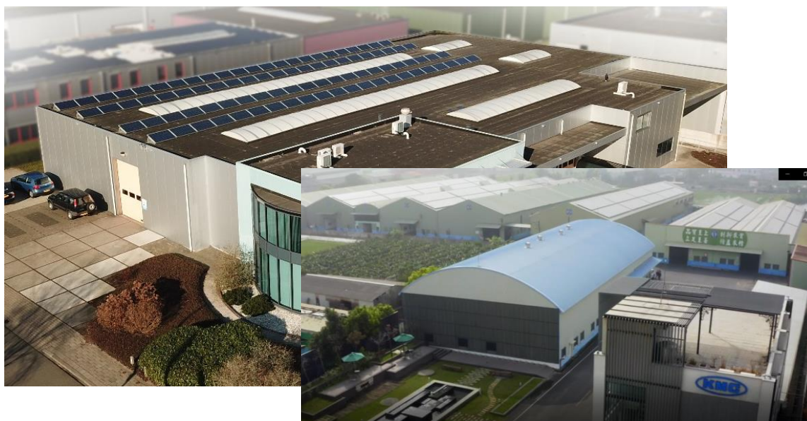
▲ The solar panels installed on the rooftop of our Taiwan and Europe company
